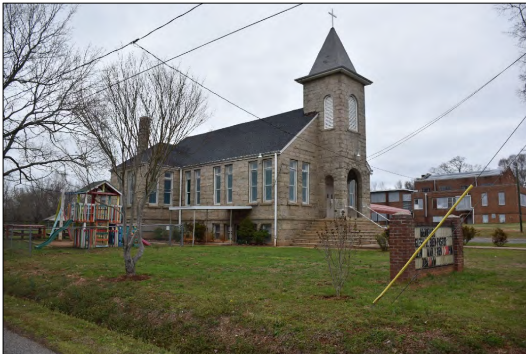
Figure 2.2.16. Rowan Mills Methodist Church, facing north.
