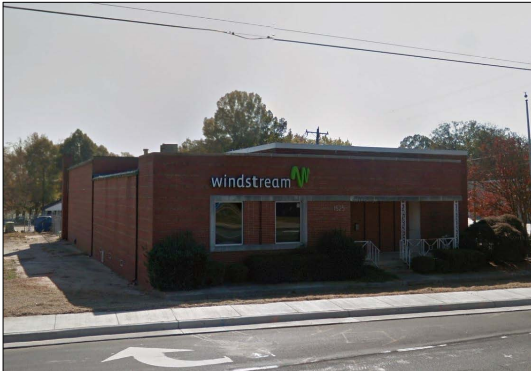
Figure 2.3.17. Concord Telephone Company Building (RW1672), facing north.
