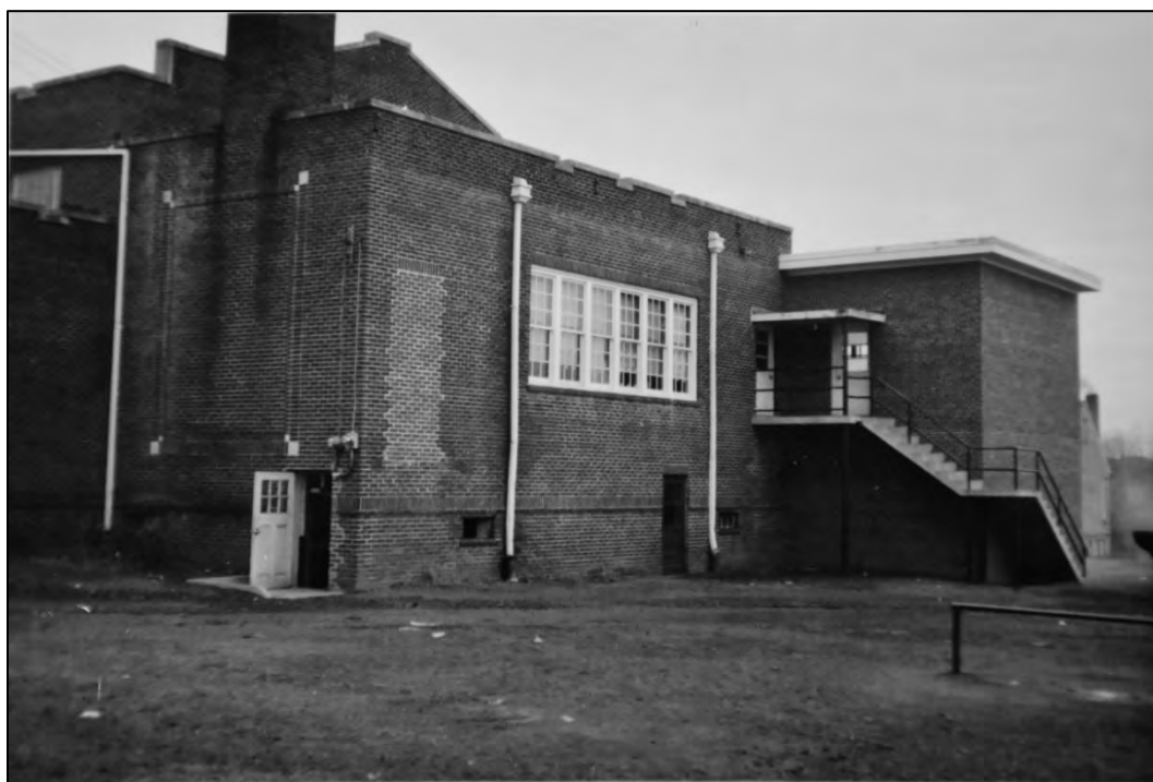
Figure 2.2.43. Photograph (undated, between 1951 and 1960) of R. G. Kizer School, rear elevation.
