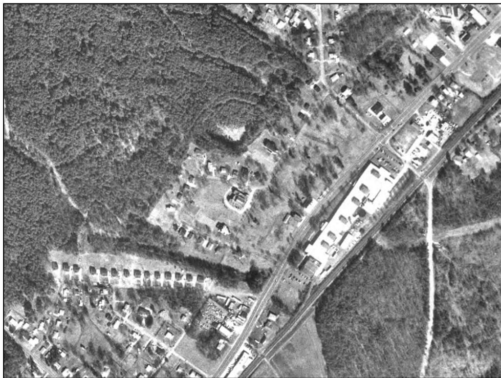
Figure 2.2.3. Aerial photograph (1993), showing the Rowan Cotton Mill complex.
