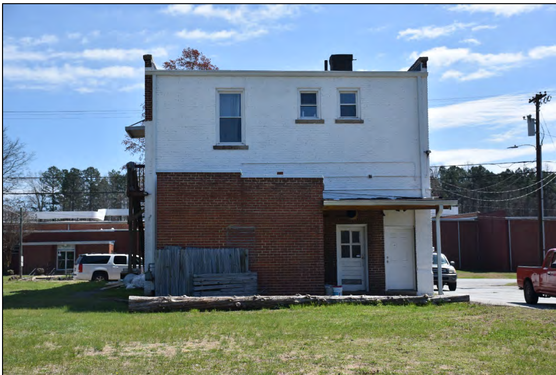
Figure 2.2.8. Rowan Mills Store, facing southeast.
