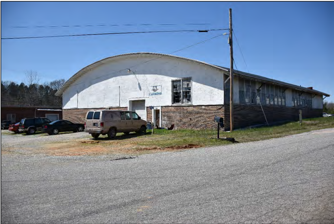
Figure 2.1.52. Salisbury Fairground Buildings, building two, facing northwest.
