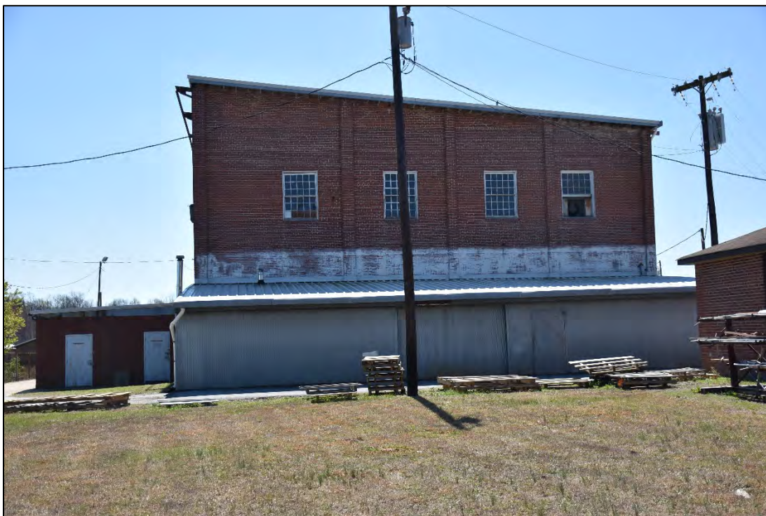
Figure 2.1.10. Salisbury Race Track Grandstand, facing south.
