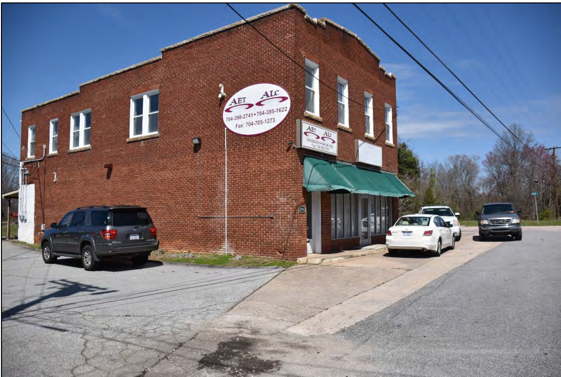
Figure 2.2.3. Rowan Mills Store (RW2181), facing north.
