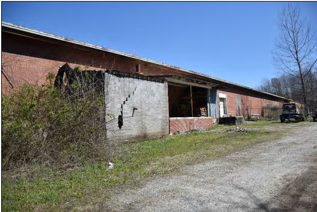
Figure 2.1.48. Salisbury Fairground Buildings, building one, facing south.
