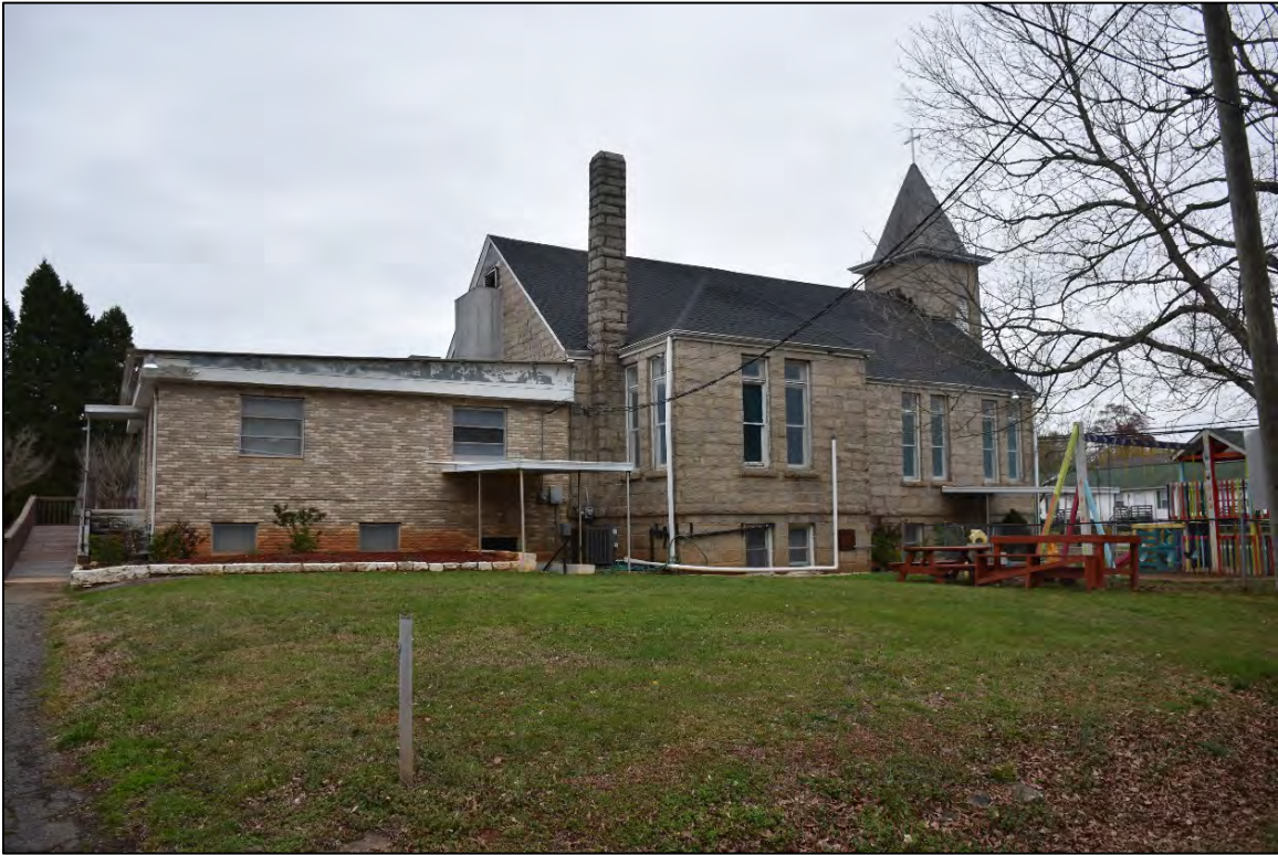
Figure 2.2.17. Rowan Mills Methodist Church, facing northeast.
