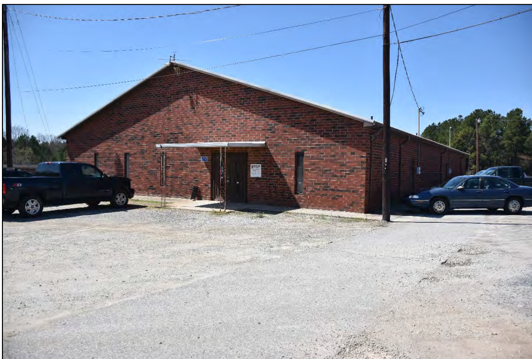
Figure 2.1.15. Salisbury Race Track Grandstand, modern office building, facing west.
