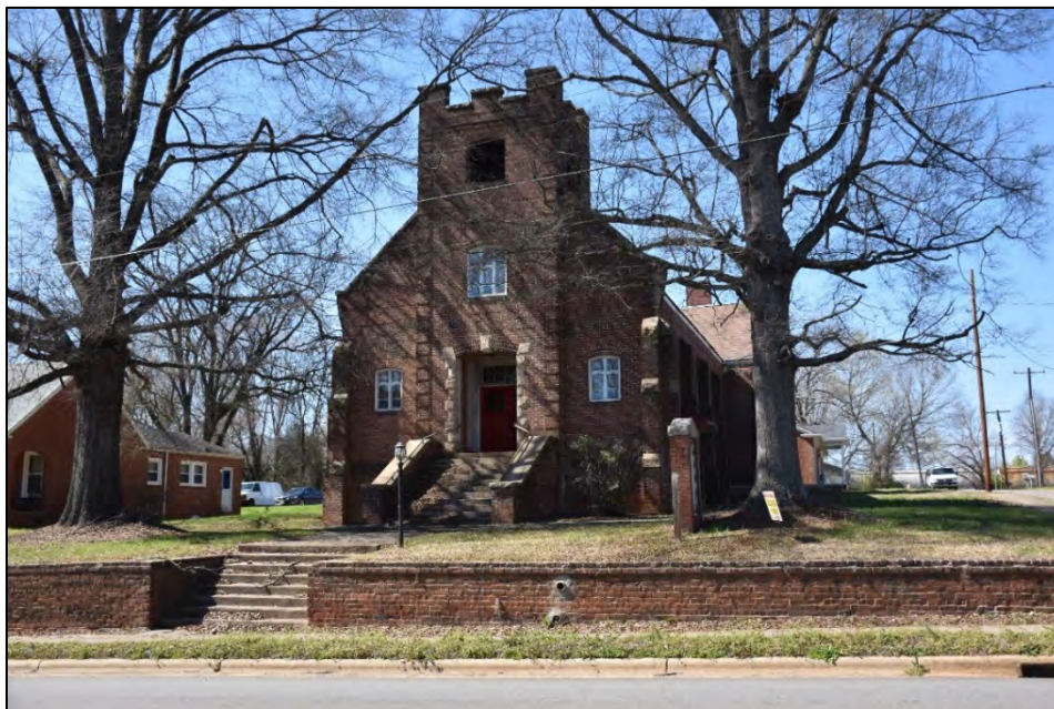
Figure 2.2.23. Christ Evangelical Lutheran Church (RW0817), facing northwest.
