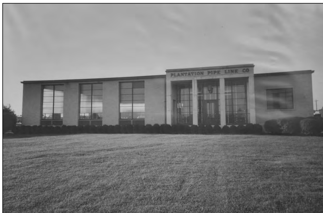
Figure 2.3.14. Undated historic photograph of the Plantation Pipe Line Pumping Station (Rowan County Library files).
