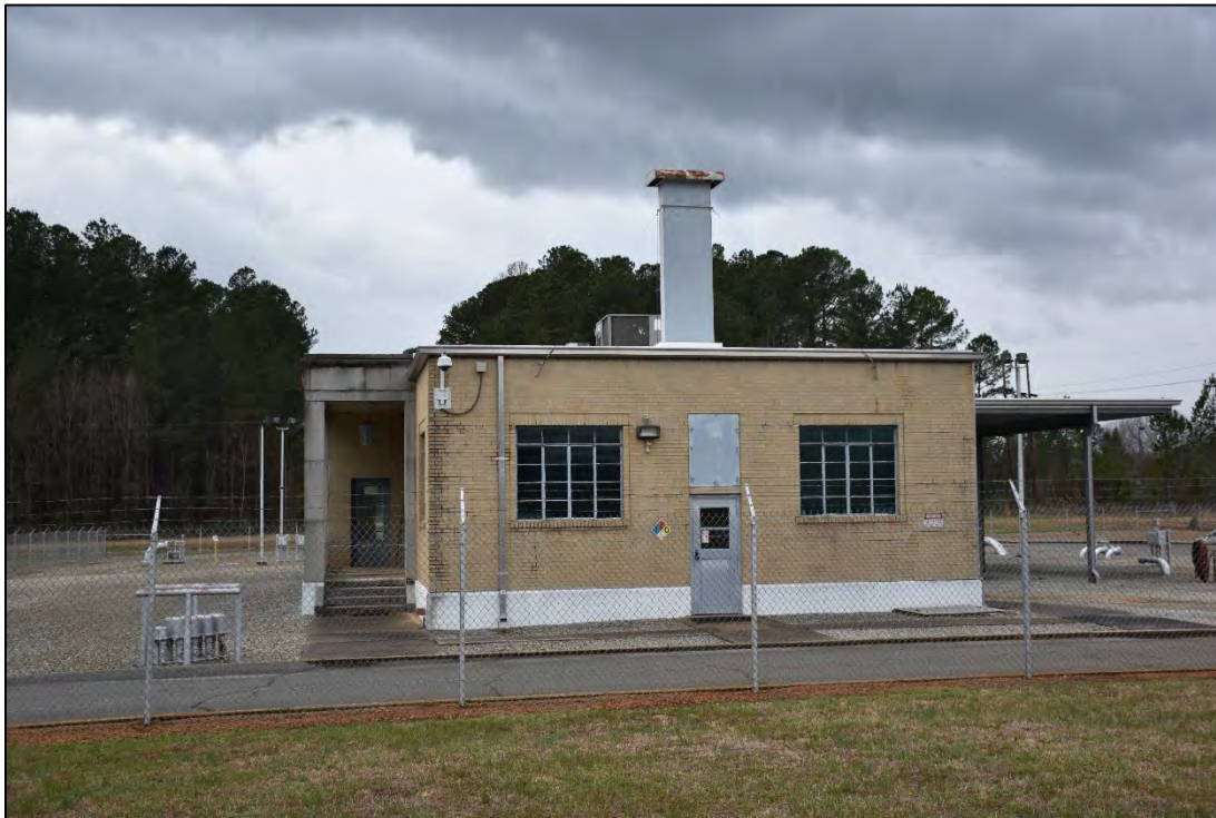
Figure 2.3.3. Plantation Pipe Line Pumping Station, facing west.
