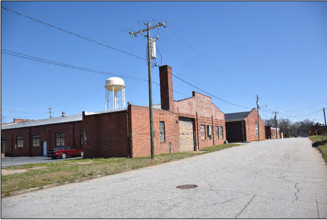
Figure 2.1.37. The Custom Furniture Company (RW1070), facing north.
