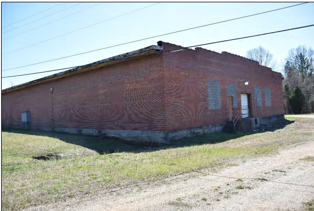
Figure 2.1.51. Salisbury Fairground Buildings, building one, facing southwest.
