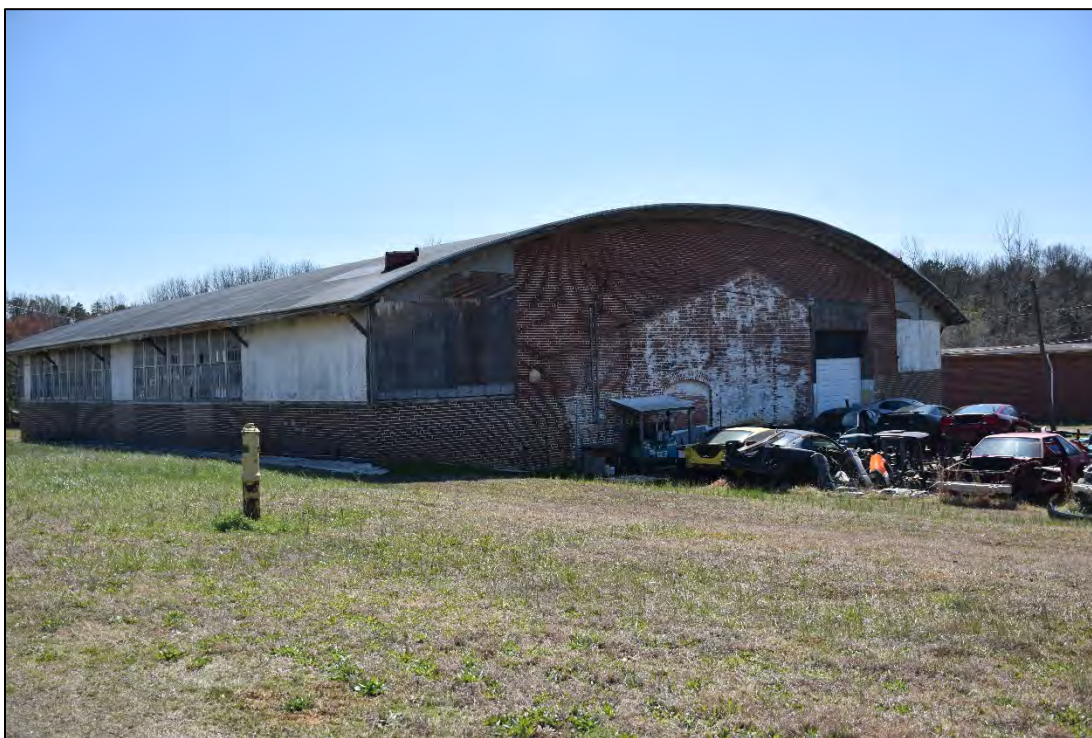
Figure 2.1.54. Salisbury Fairground Buildings, building two, facing south.
