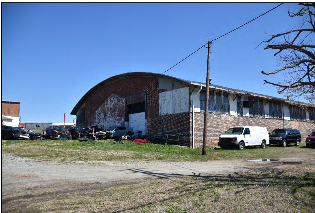
Figure 2.1.56. Salisbury Fairground Buildings, building two, facing east.
