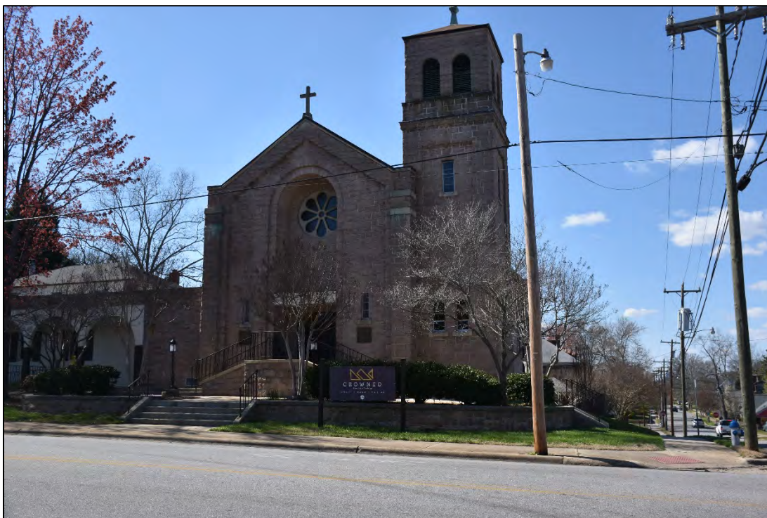
Figure 2.2.25. Church, 124 North Fulton Street (RW1970), facing northwest.
