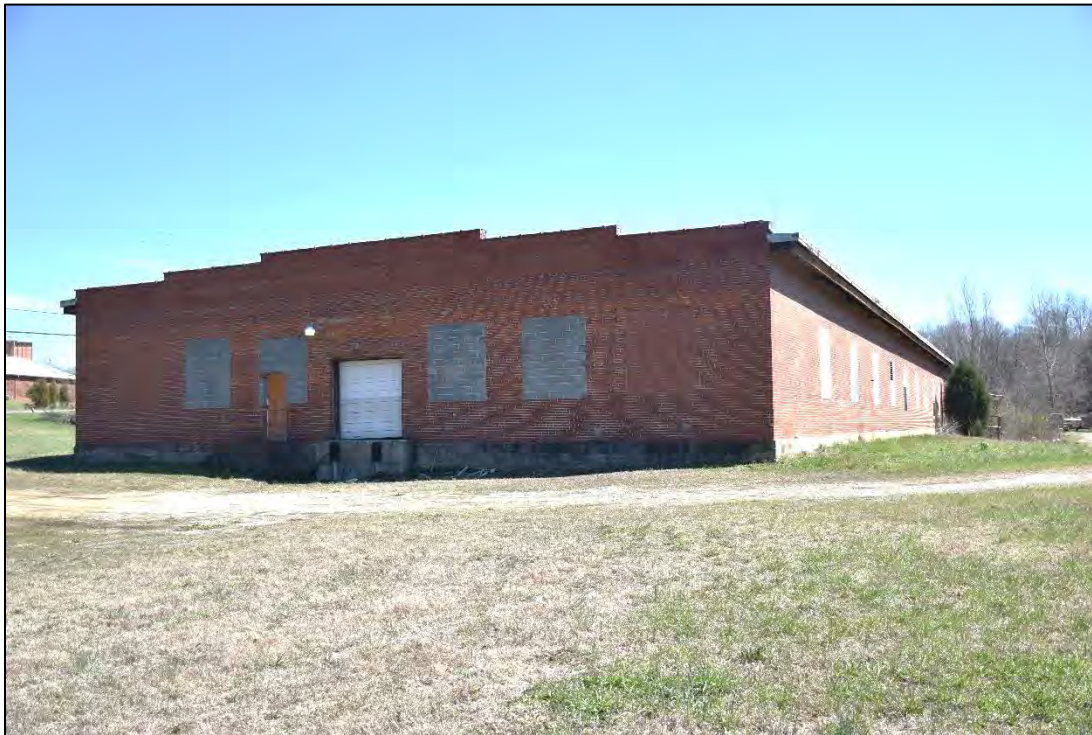
Figure 2.1.50. Salisbury Fairground Buildings, building one, facing east.
