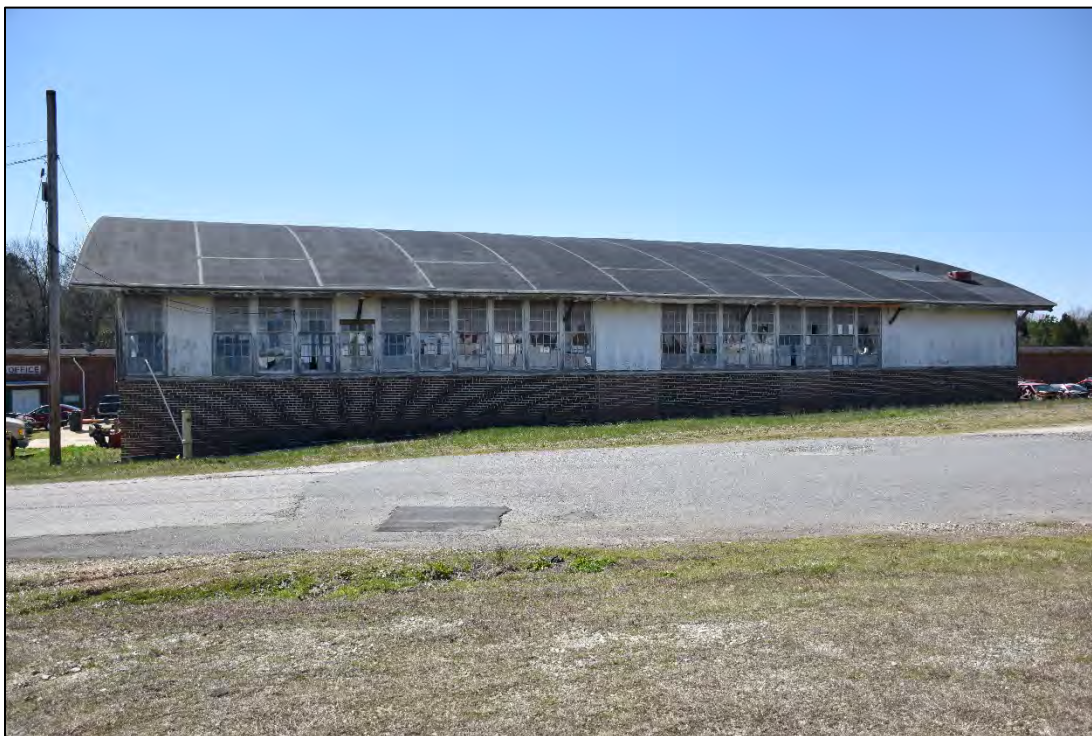
Figure 2.1.53. Salisbury Fairground Buildings, building two, facing west.
