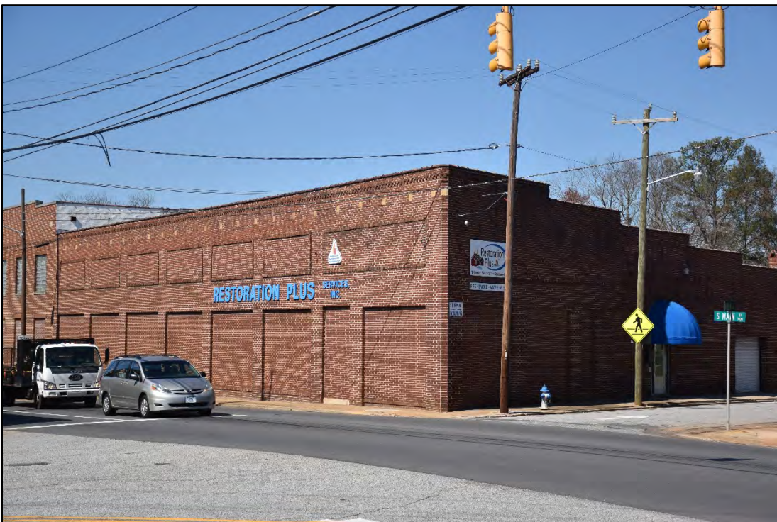
Figure 2.1.68. Stanback Warehouses (RW1465), facing northwest.
