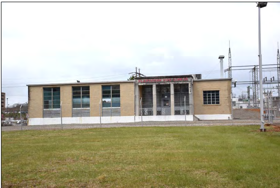
Figure 2.3.1. Plantation Pipe Line Pumping Station (RW2185), facing north.
