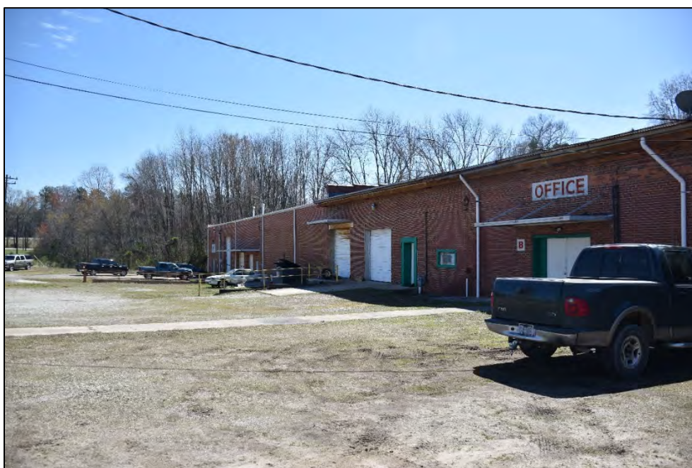
Figure 2.1.40. Salisbury Fairground Buildings, building one, facing south.
