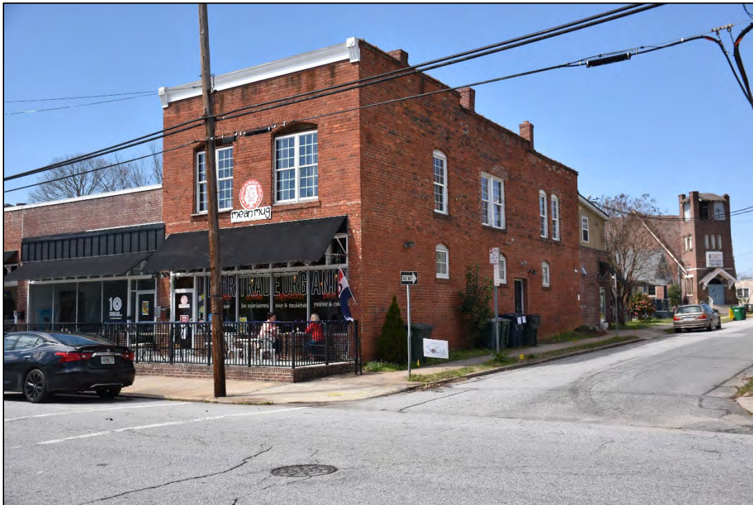
Figure 2.2.12. The (former) R. L. Foil Grocery (RW1466), facing southwest.
