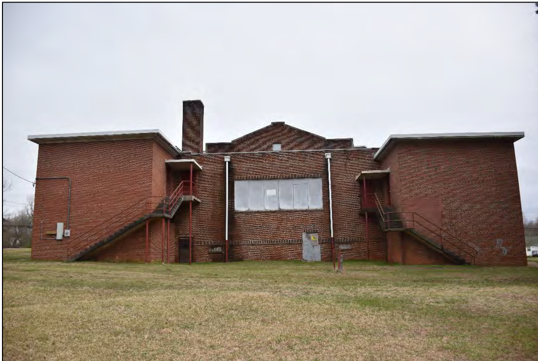
Figure 2.2.32. R. G. Kizer School, facing southeast.
