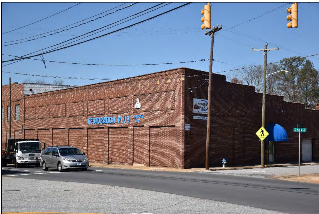
Figure 2.1.34. Stanback Warehouses (RW1465), facing northwest.
