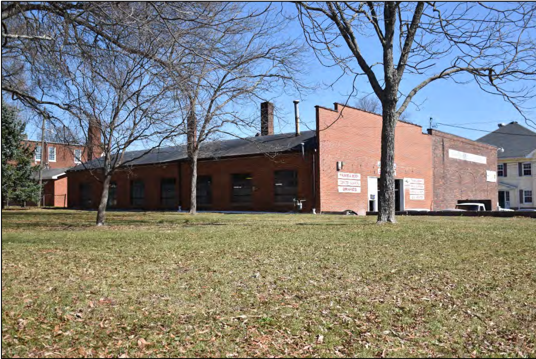
Figure 2.1.67. Jackson Alignment/Jack Kepley Scout Building (RW2104), facing northeast.
