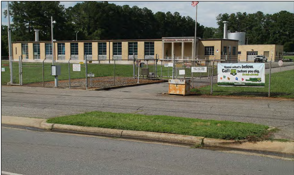
Figure 2.3.15. Plantation Pipe Line Pumping Station in Lowell (NSN), facing northeast.
