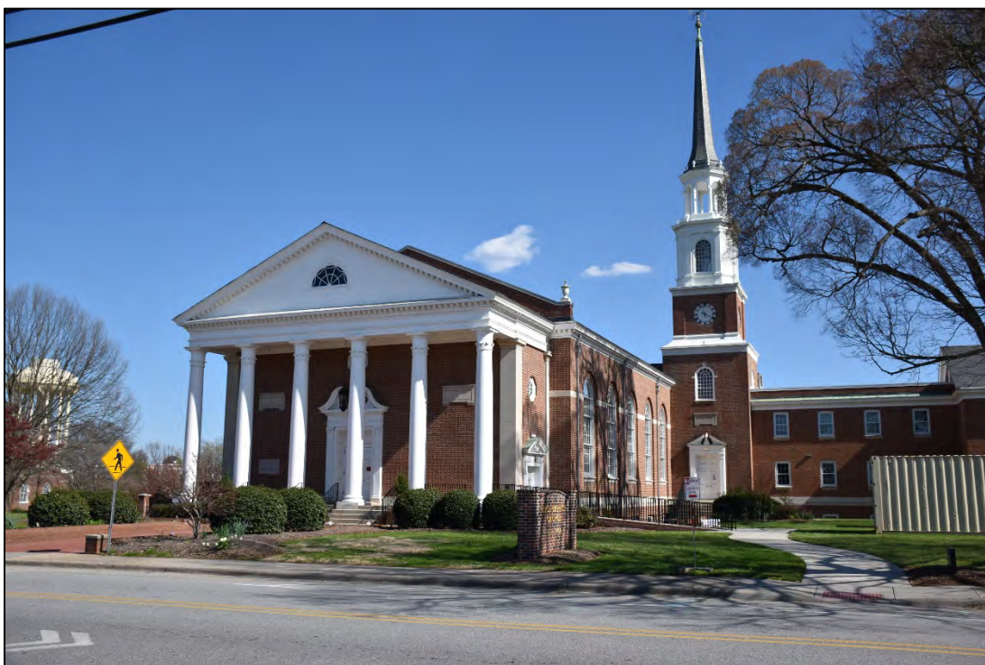
Figure 2.2.60. First Baptist Church (RW0962), facing southeast.
