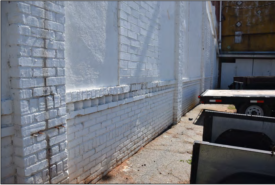
Figure 2.1.4. Salisbury Race Track Grandstand, brick detail along west wall, facing south.
