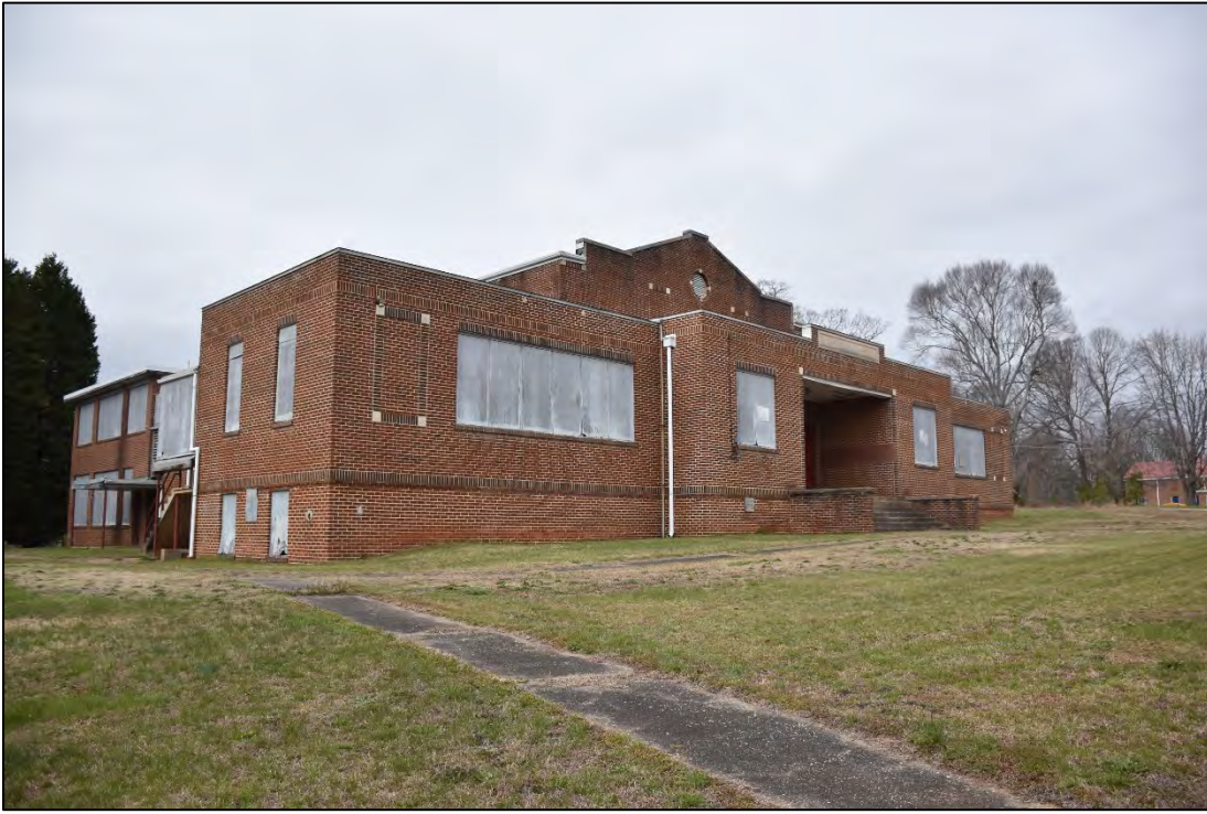
Figure 2.2.29. R. G. Kizer School, facing north.
