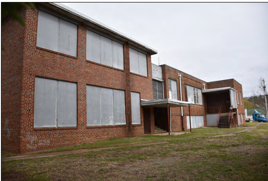
Figure 2.2.31. R. G. Kizer School, facing east.
