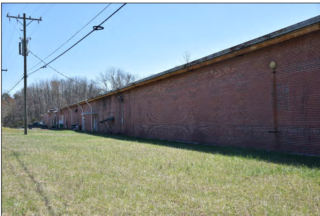
Figure 2.1.44. Salisbury Fairground Buildings, building one, facing south.
