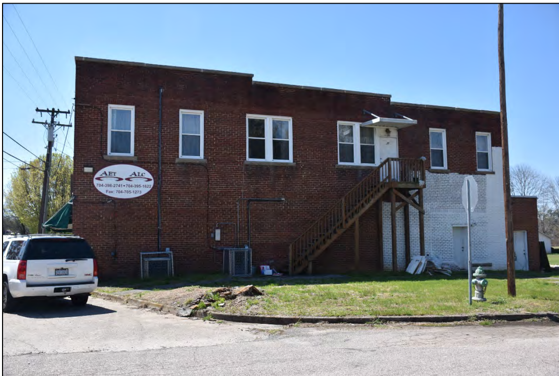
Figure 2.2.6. Rowan Mills Store, facing southwest.
