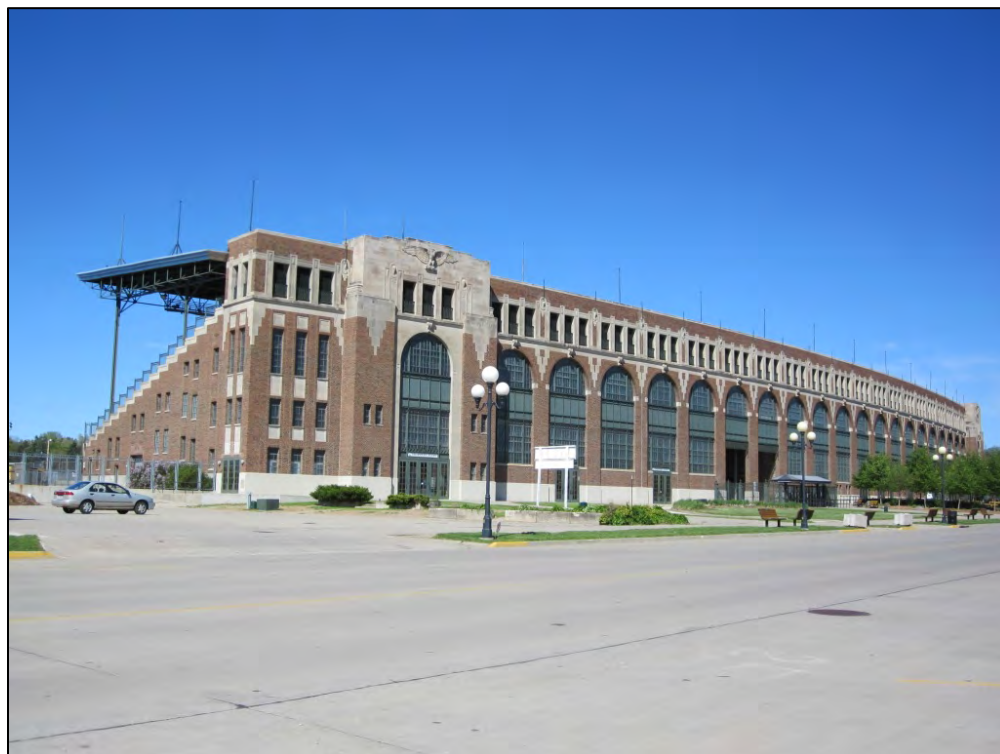
Figure 2.1.31. Iowa State Fairgrounds Grandstand, built circa-1930s.
