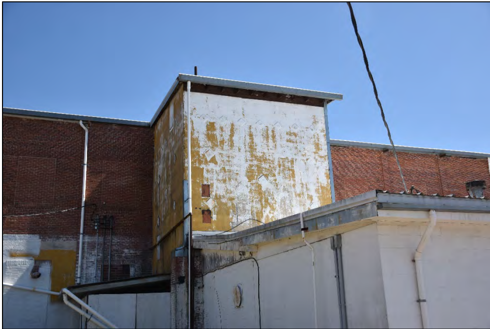
Figure 2.1.2. Salisbury Race Track Grandstand, tower, facing east.
