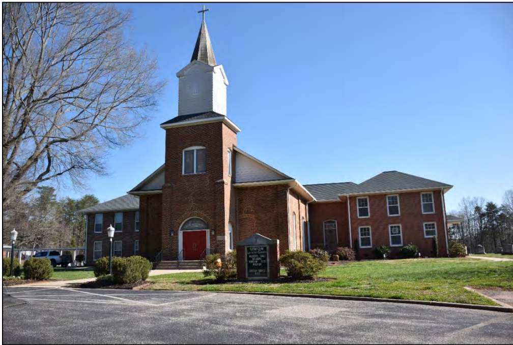
Figure 2.2.24. Union Evangelical Lutheran Church (RW0754), facing northeast.
