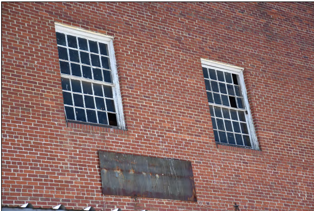
Figure 2.1.8. Salisbury Race Track Grandstand, window detail, facing northwest.
