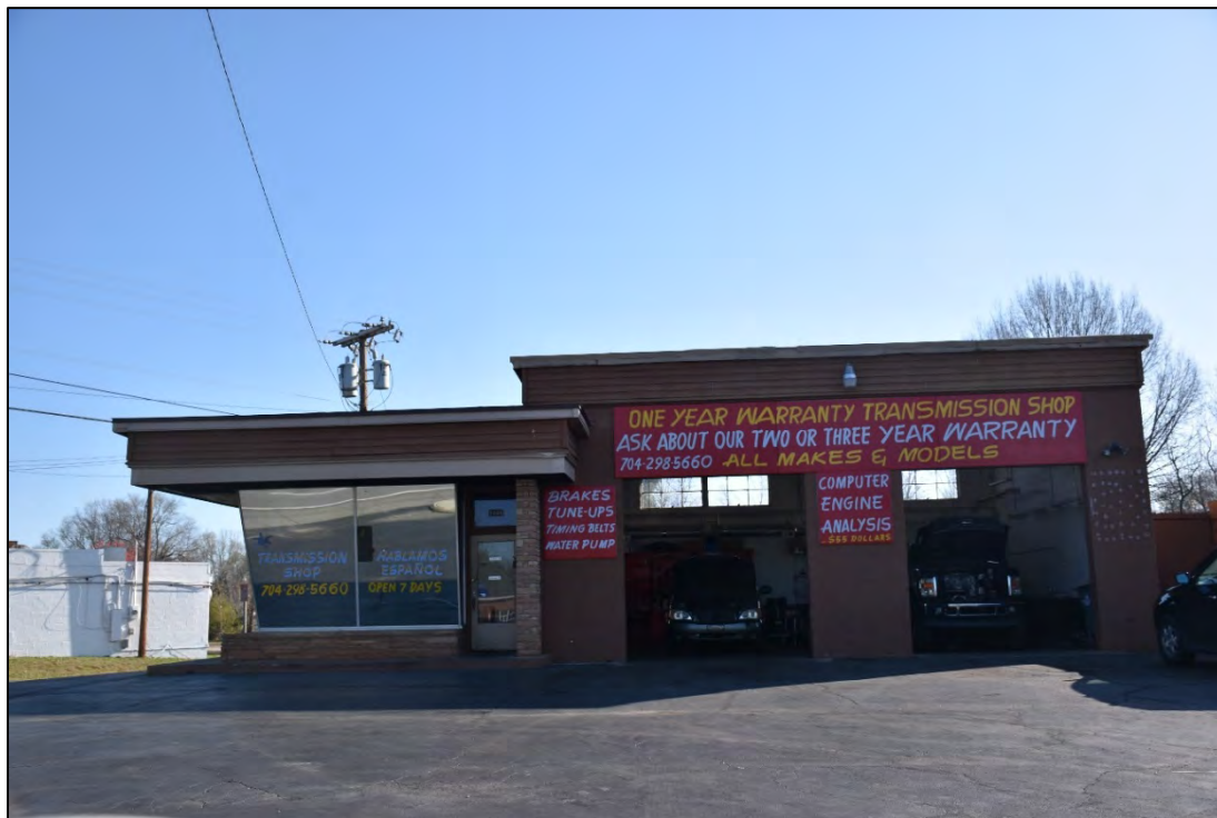
Figure 2.3.16. Gas station (RW1647), facing northeast.
