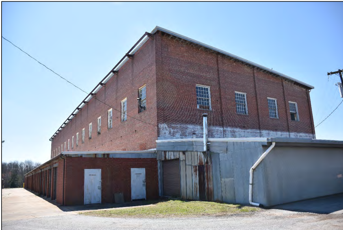
Figure 2.1.9. Salisbury Race Track Grandstand, facing southwest.
