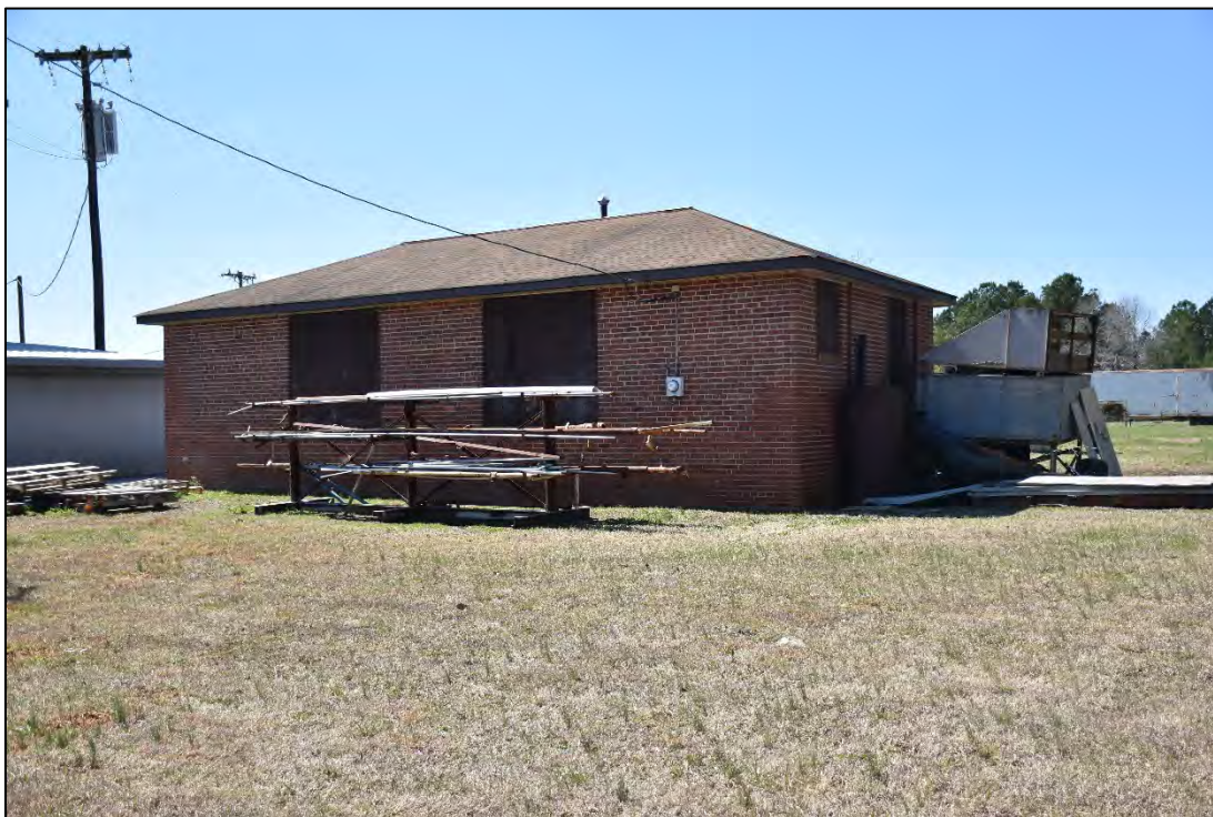
Figure 2.1.12. Salisbury Race Track Grandstand, concession stand, facing southwest.
