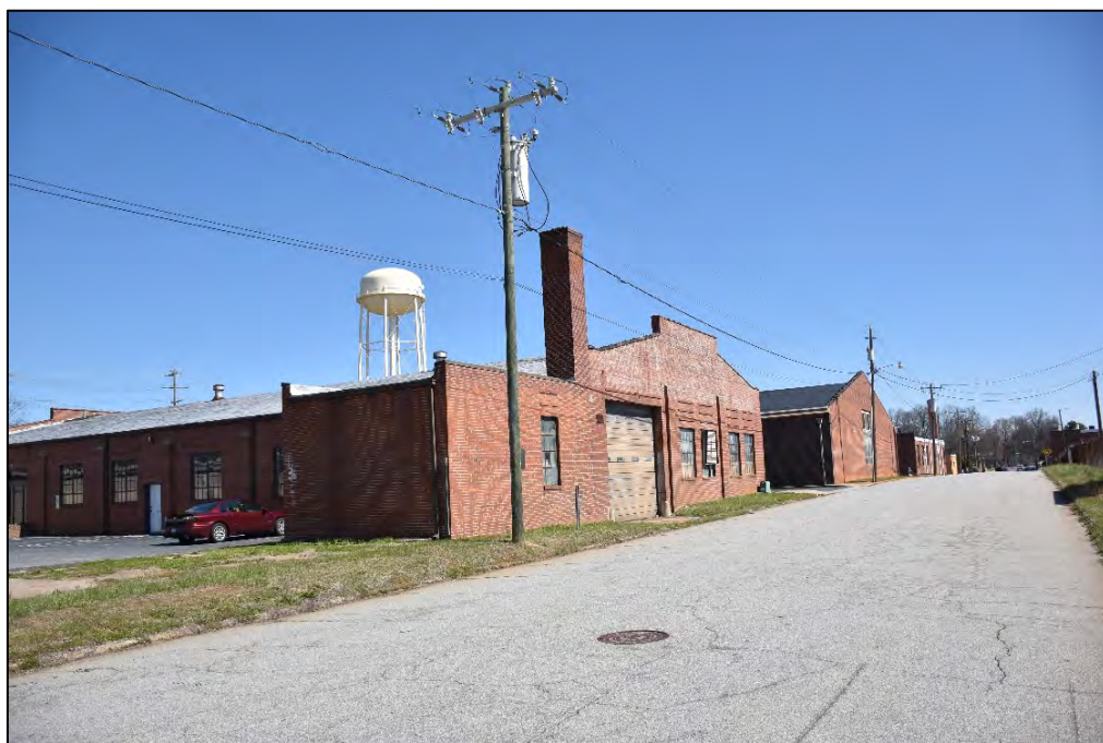
Figure 2.1.66. The Custom Furniture Company (RW1070), facing north.
