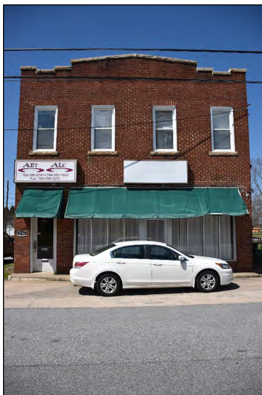
Figure 2.2.4. Rowan Mills Store, facing northwest.
