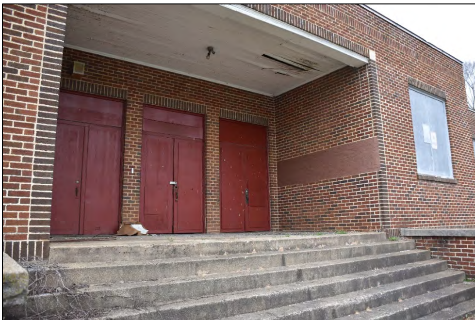
Figure 2.2.28. R. G. Kizer School, entry detail, facing north.
