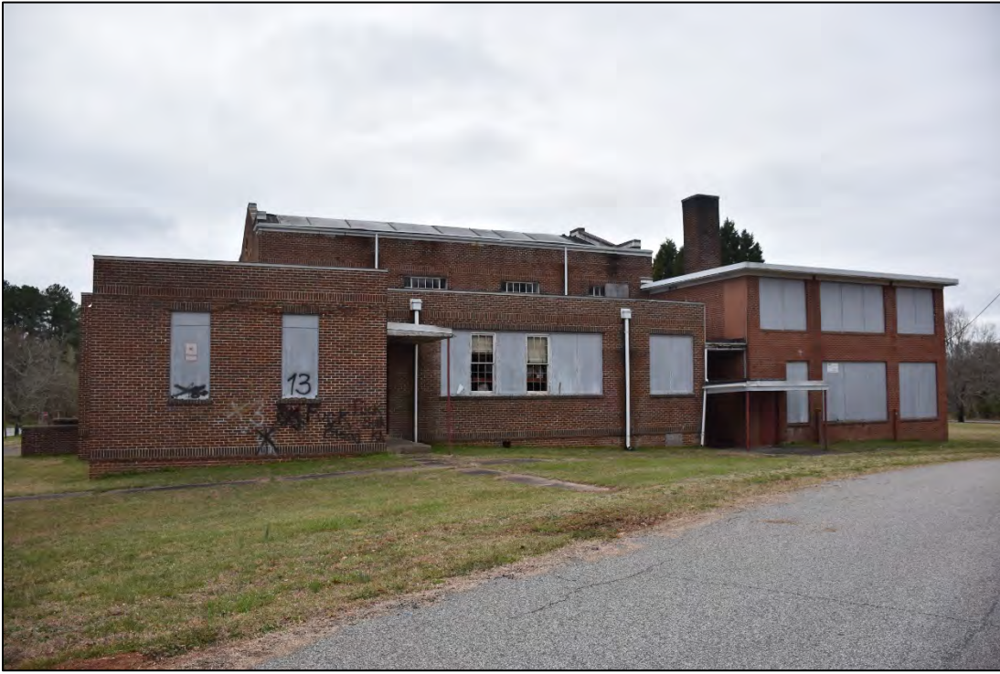
Figure 2.2.34. R. G. Kizer School, facing southwest.
