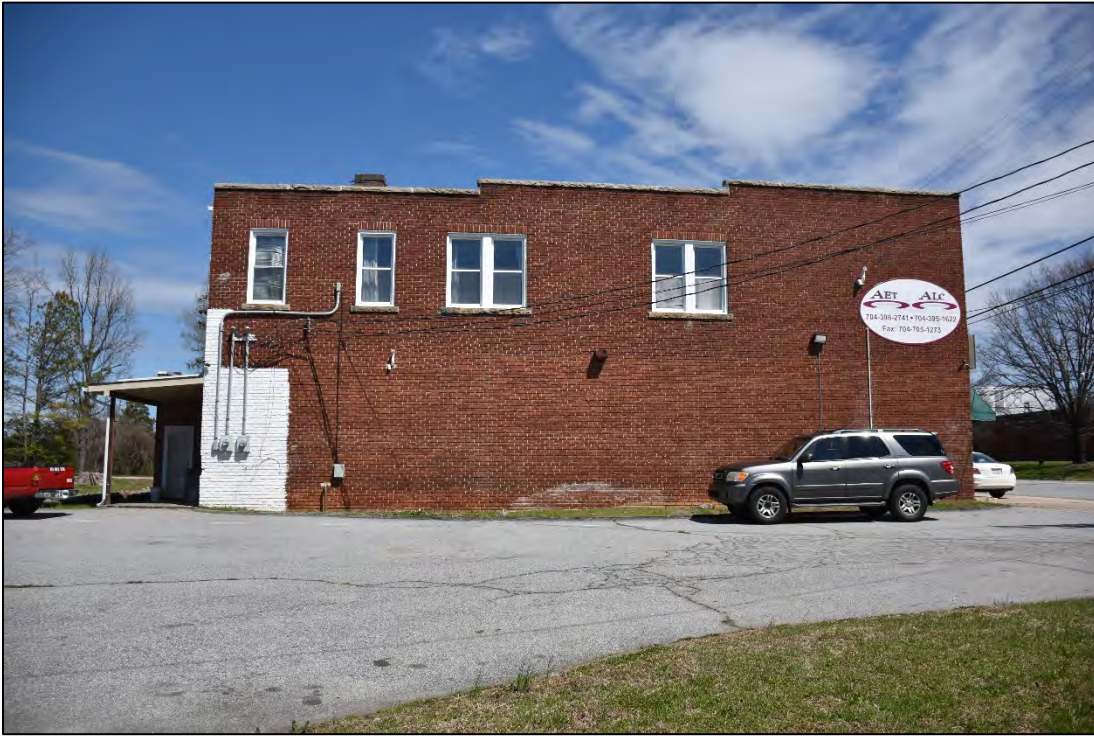
Figure 2.2.9. Rowan Mills Store, facing northeast.
