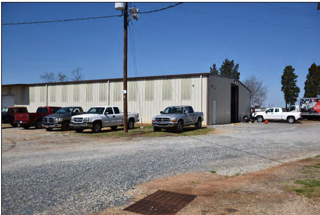
Figure 2.1.14. Salisbury Race Track Grandstand, metal storage building, facing northwest.
