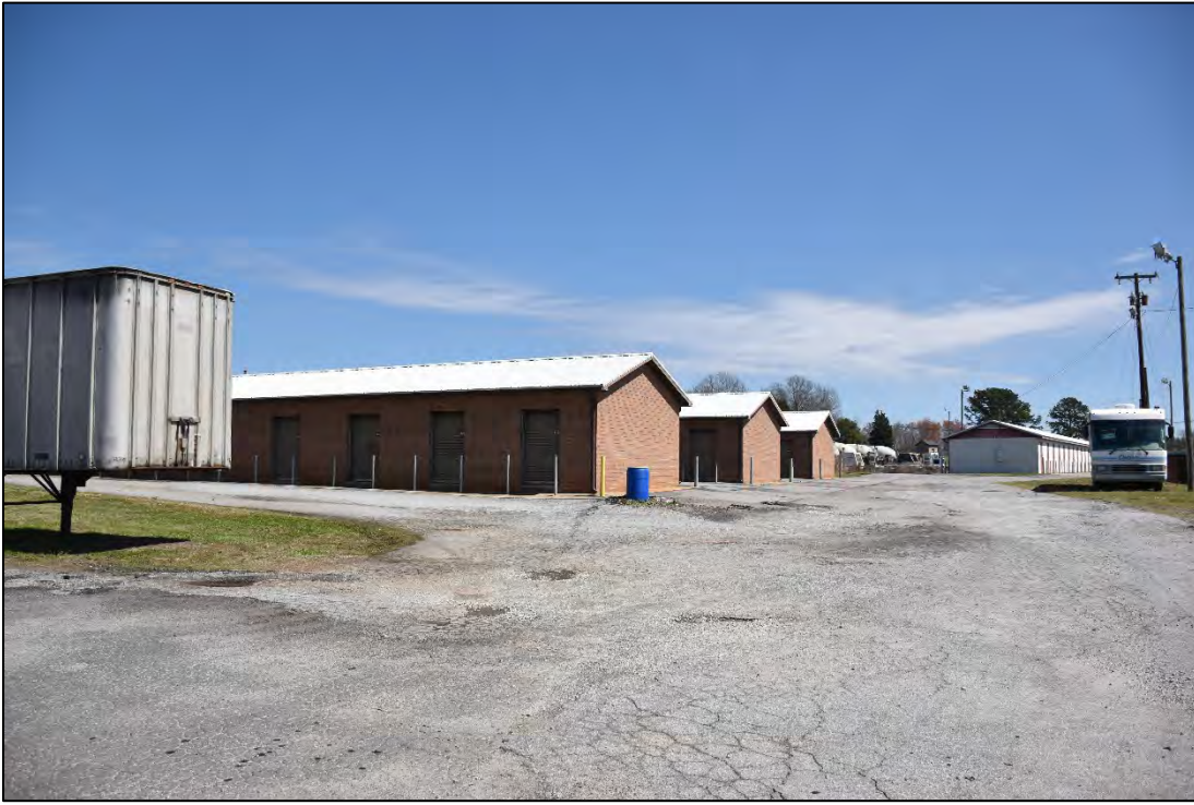
Figure 2.1.16. Salisbury Race Track Grandstand, modern storage buildings, facing east.
