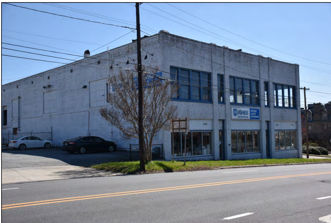
Figure 2.1.36. Hughes Southeastern Building (RW2103), facing south.
