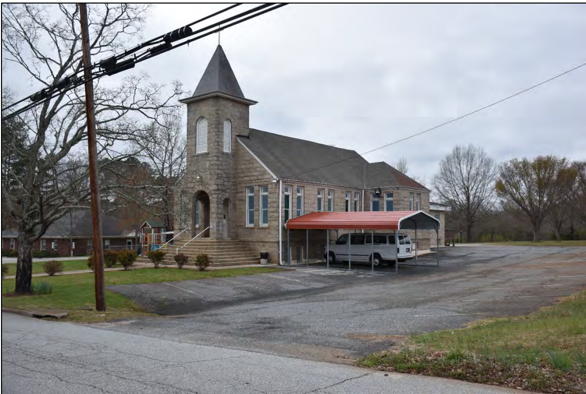
Figure 2.2.14. Rowan Mills Methodist Church (RW2182), facing west.
