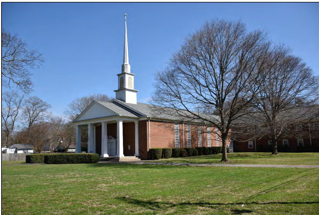
Figure 2.2.58. North Main Baptist Church (RW0168), circa 1960, facing southeast.
