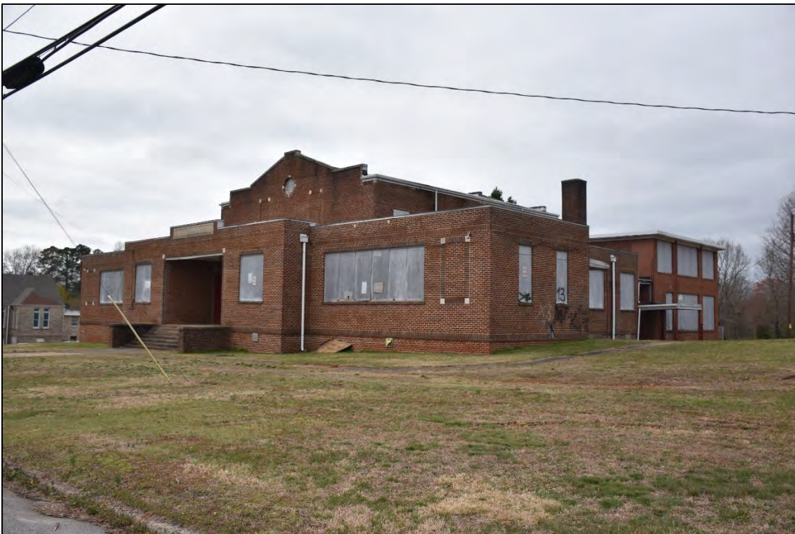
Figure 2.2.26. R. G. Kizer School (RW2183), facing west.
