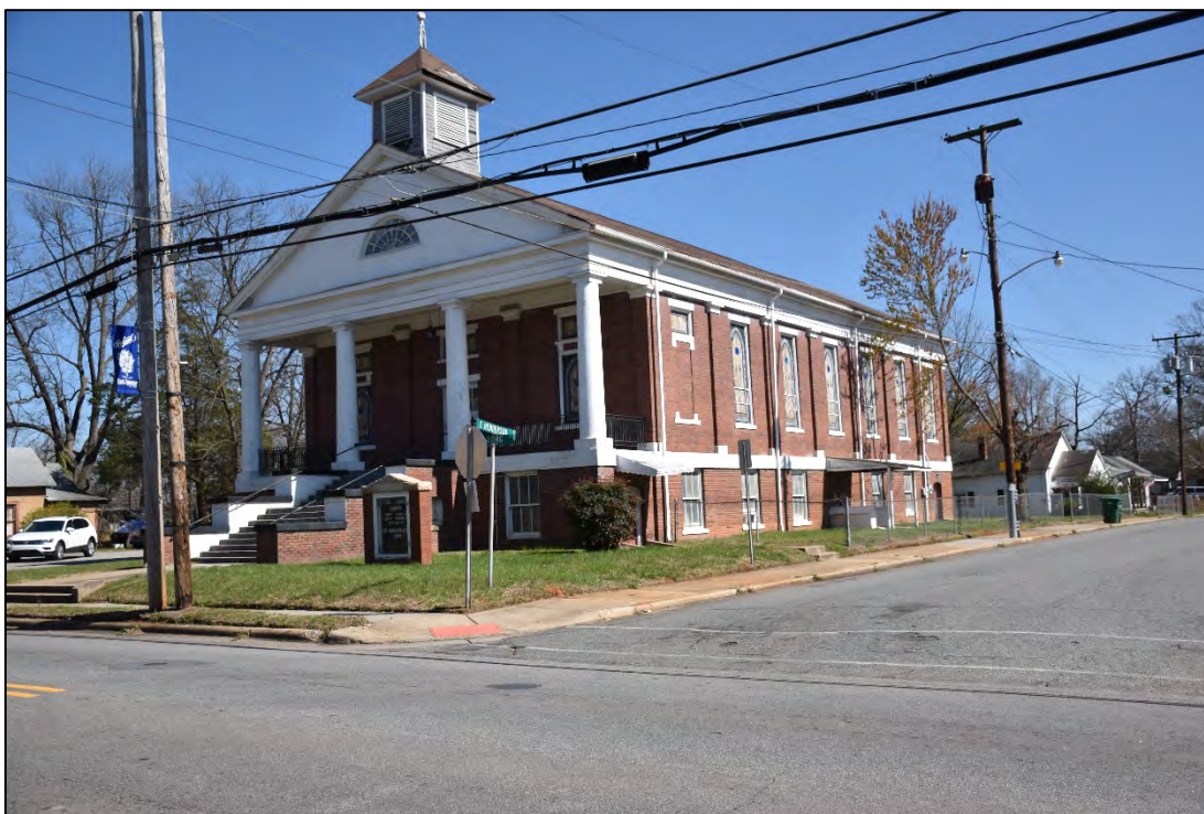
Figure 2.2.59. Long Street Methodist Episcopal Church (NSN), built 1920, facing southeast.
