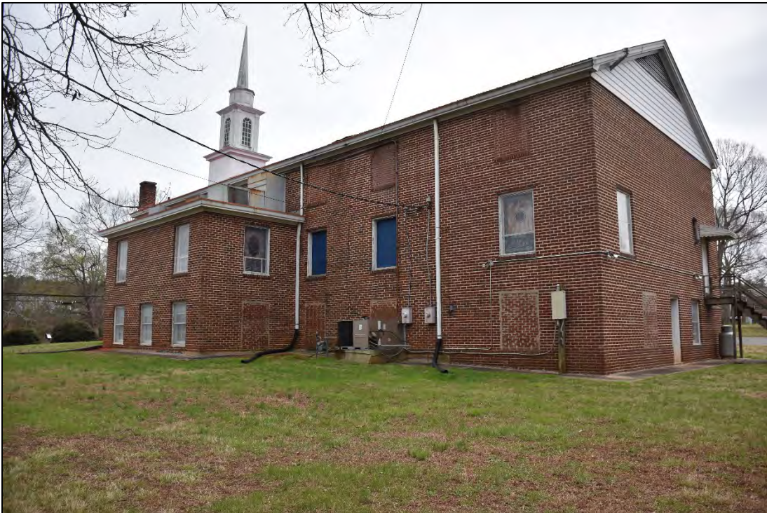
Figure 2.2.51. Rowan Mills Baptist Church, facing south.
