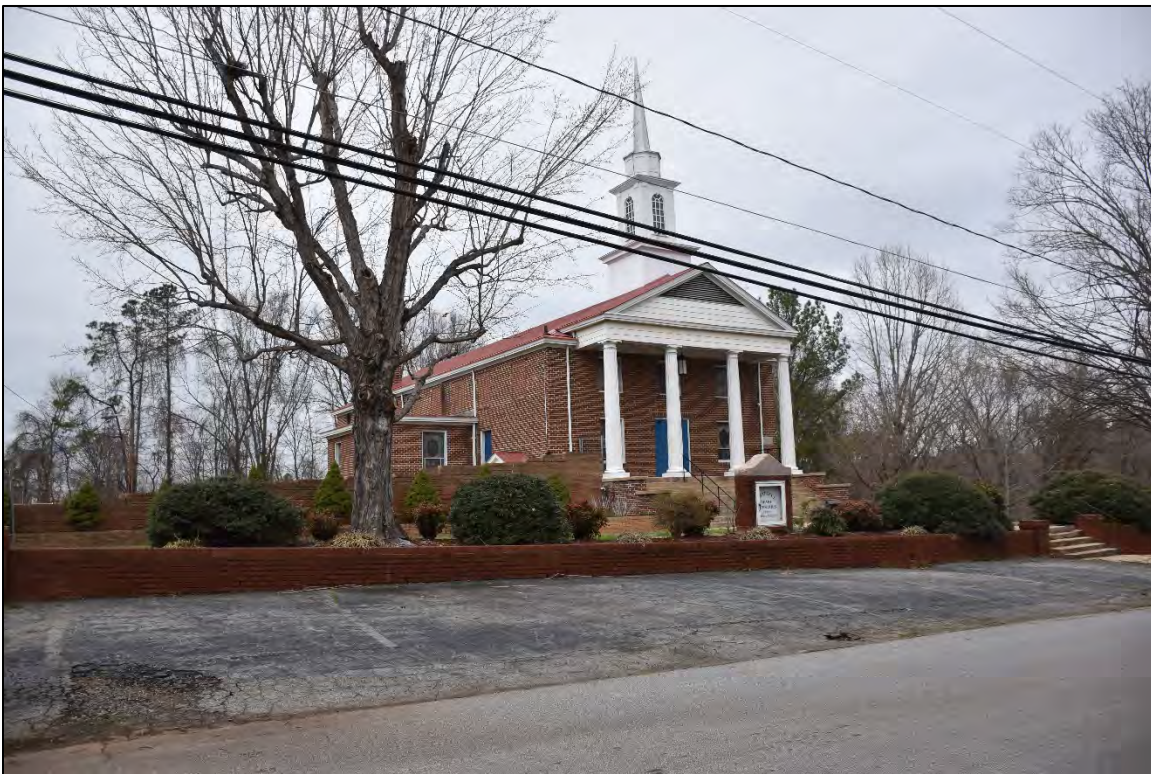
Figure 2.2.48. Rowan Mills Baptist Church (RW2184), facing north.
