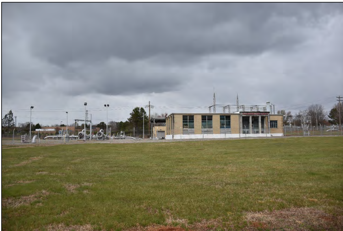
Figure 2.3.8. Plantation Pipe Line Pumping Station, facing north.
