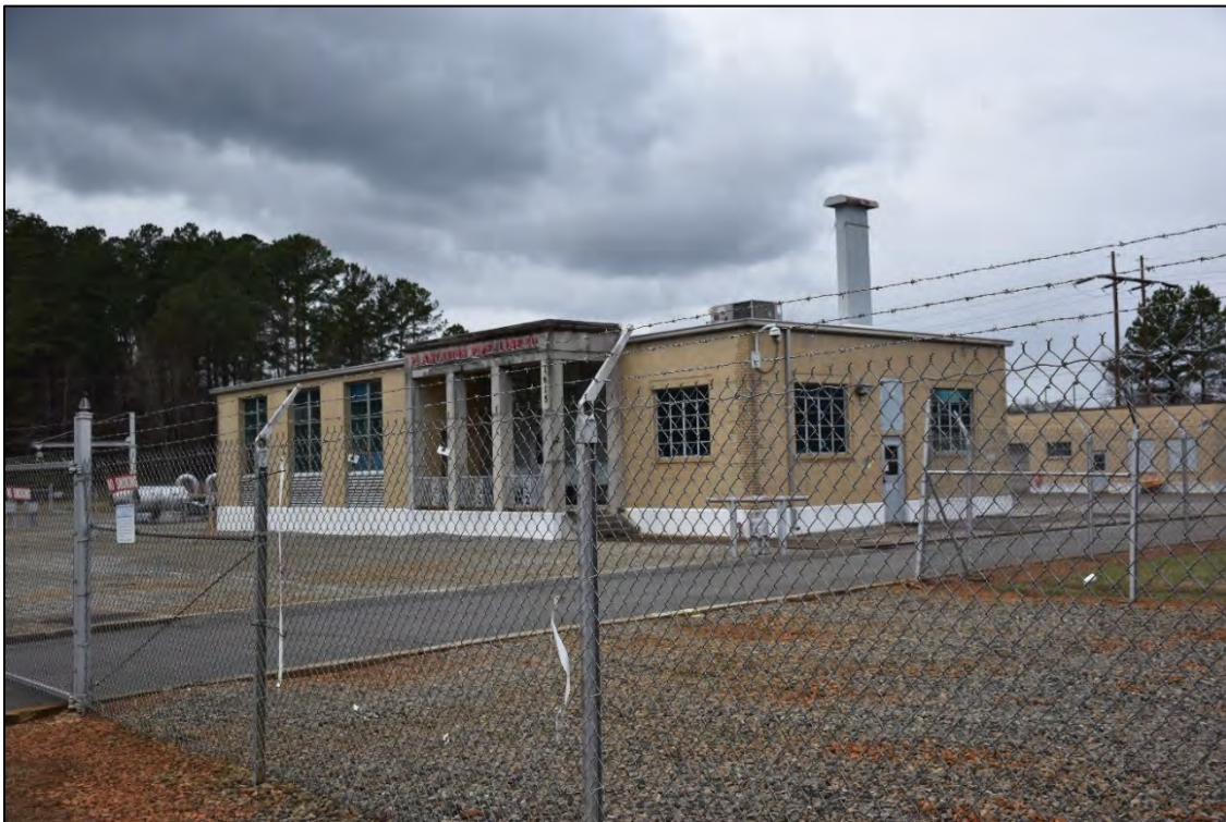
Figure 2.3.2. Plantation Pipe Line Pumping Station, facing northwest.
