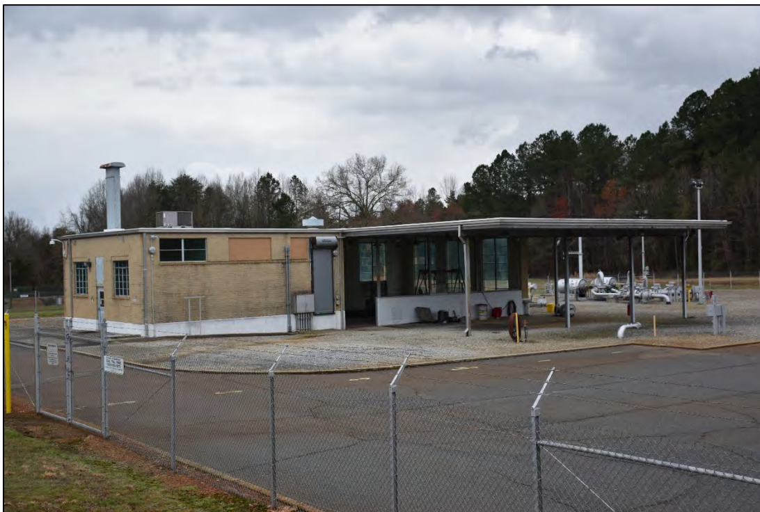
Figure 2.3.4. Plantation Pipe Line Pumping Station, facing southwest.
