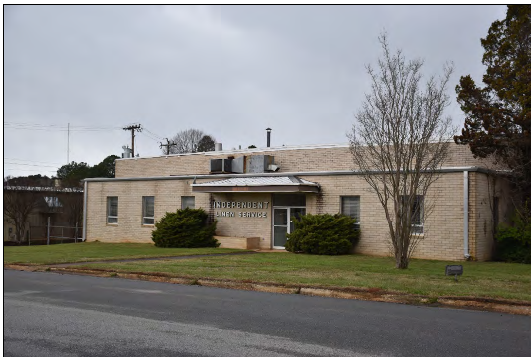
Figure 2.3.18. Independent Linen Service building (NSN), facing north.
