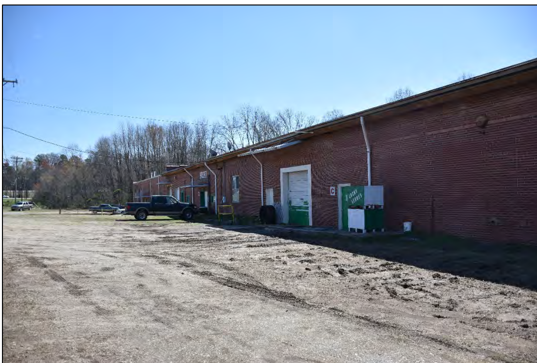
Figure 2.1.42. Salisbury Fairground Buildings, building one, facing south.
