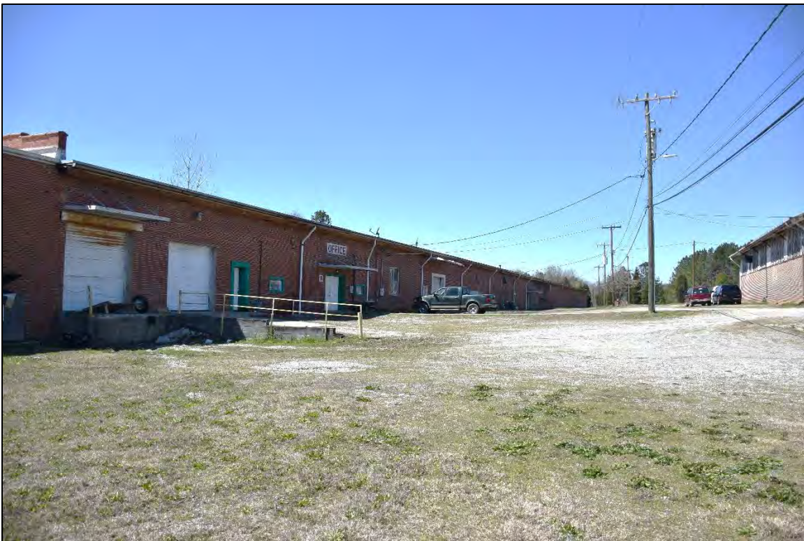
Figure 2.1.38. Salisbury Fairground Buildings (RW2180), facing northwest.
